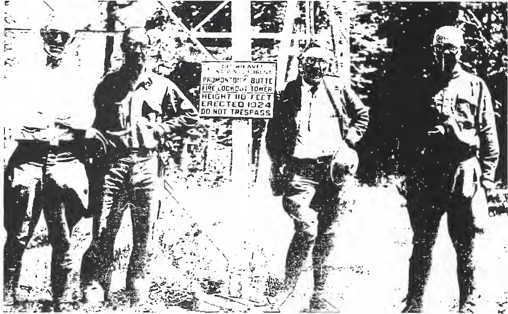
Figure 18. Promontory Fire Tower, Sitgreaves National Forest, September 1928.
